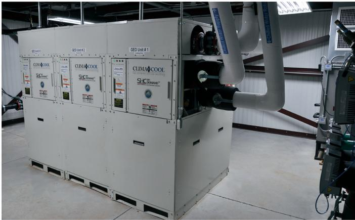
According to Darrin Beller, president of Air Products Supply, this ClimaCool configuration incorporates several notable features that maintain precise chilled and hot water temperatures, building loads and compressor run time equalization for ultimate operational efficiency.
