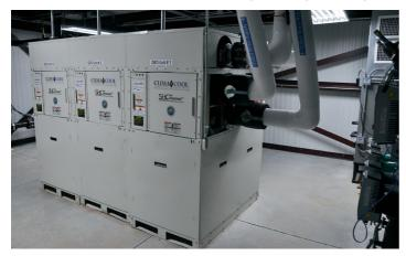
According to Darrin Beller, president of Air Products Supply, this ClimaCool configuration incorporates several notable features that maintain precise chilled and hot water temperatures, building loads and compressor run time equalization for ultimate operational efficiency.
